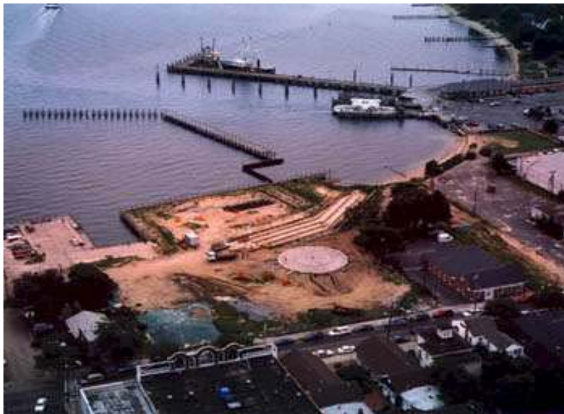
The site during construction
