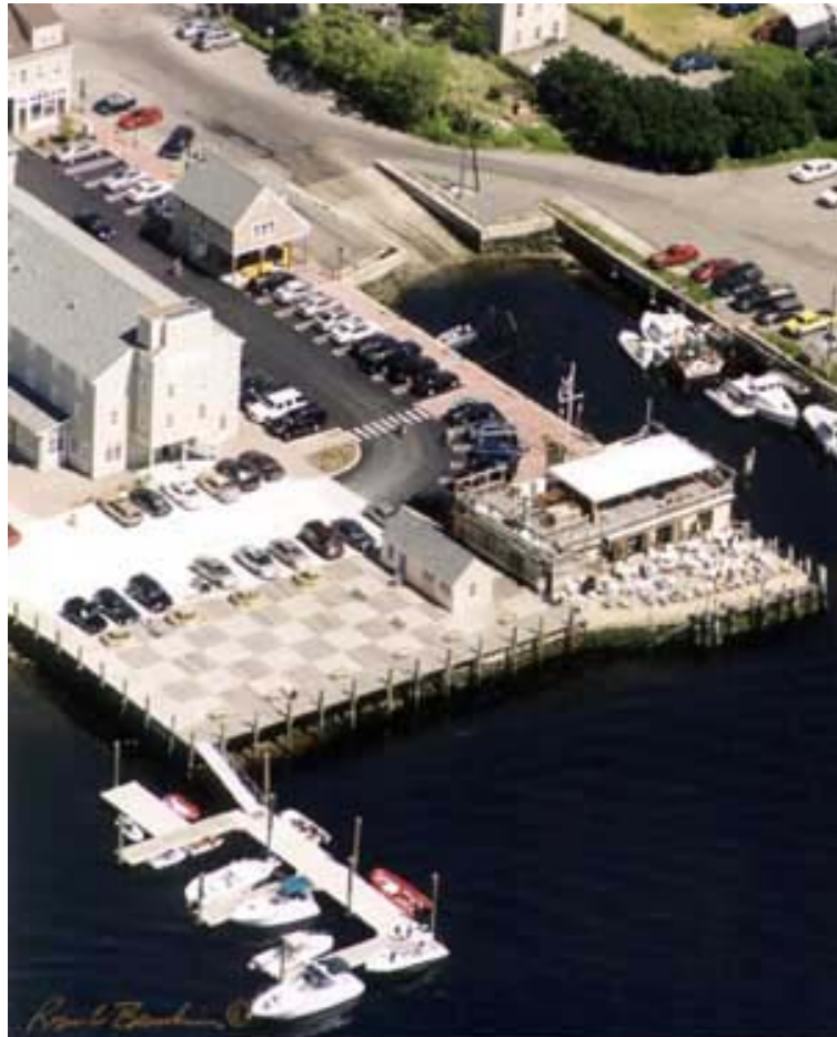
Thames Street Landing after Construction
